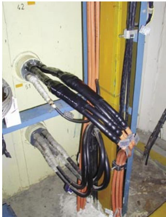
Cable joints made by Kabelovna KABEX® a.s. as used on a bushing wall in NPP Dukovany
